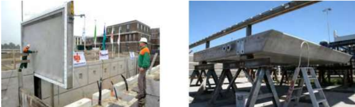
Figure 38: UHPFRC water lock gate construction, source: (Cement, 2013)
