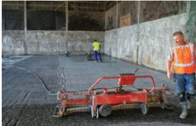
Figure 34: industrial UHPFRC floor at waste recycling sorting plant, source: (Buitelaar, 2018)
