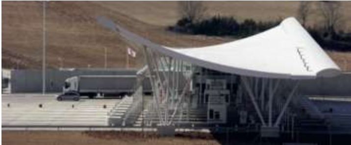
Figure 33: thin roof of toll station in Millau, source: (Berendsen, 2014)
