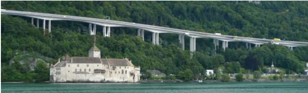
Figure 27: Chillon viaducts in Switzerland, source: (Brühwiler, et al., 2015)
