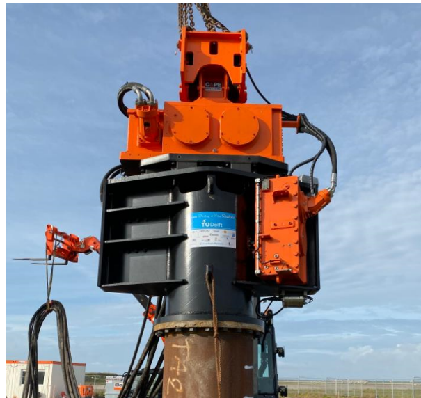
Figure 1: The GDP shaker connected to a pile via a bolted flange connection.
