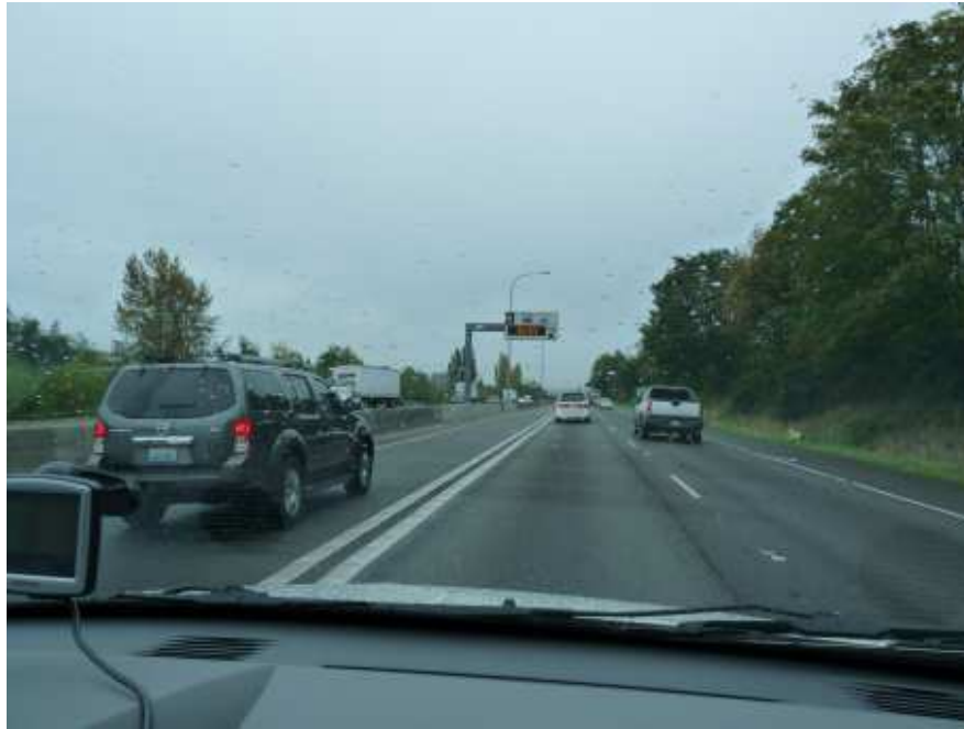
Figure 18: HOT Lane in Seattle
