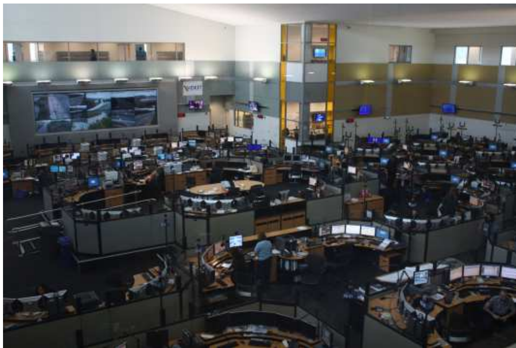
Figure 8: VDOT Traffic Control Center
