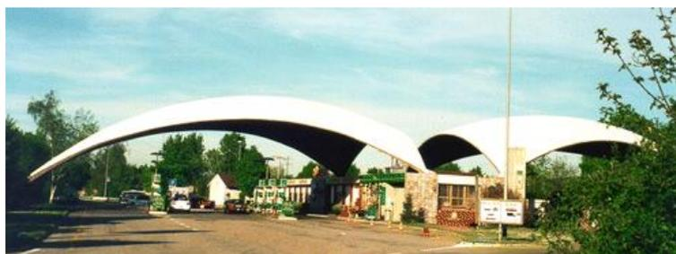
Figure 2.1: Thin concrete shell covering a service station near Deitingen by Heinz Isler (Photo: Eugen Brühwiler)
