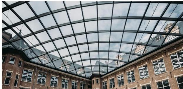
Figure 2.3: C30 Shell grid shell structure © Octatube, 2022
