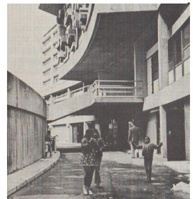
10 Inside the sunken driveway
