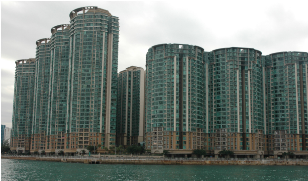
Figure 1. Concentrated high-rise development in Hong Kong, China.
