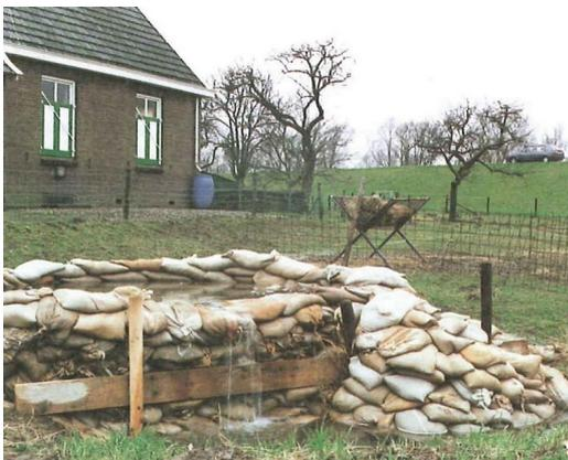
Figure 1.3: Internal erosion (TAW, 1995)
