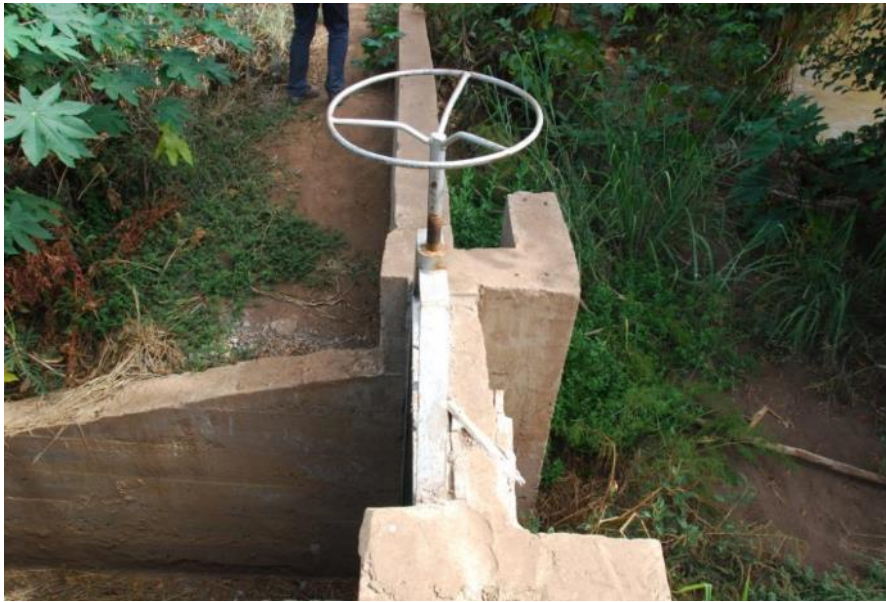
Figure 123: Erosion at the existing spillway, observed during fieldwork 1
