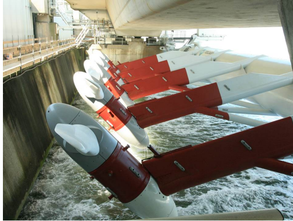
Figure 1.2: Photo of a gate of the Dutch storm surge barrier with five tidal turbines (here: the turbines are parked above the water and not in operation).
