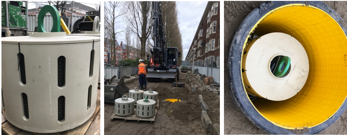
Figure C - 2: Installation of SediSorp+ cartridges in S3
