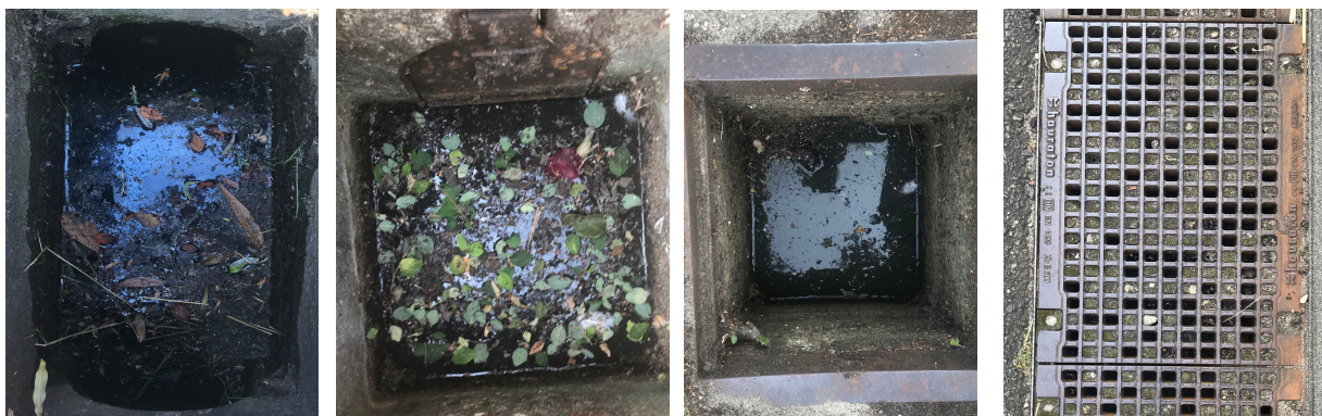
Figure C - 11: Gully pots and line gutter at the locations along the Loosdrecht horseshoe road monitored by Mandemakers and Holsteijn in 2018
