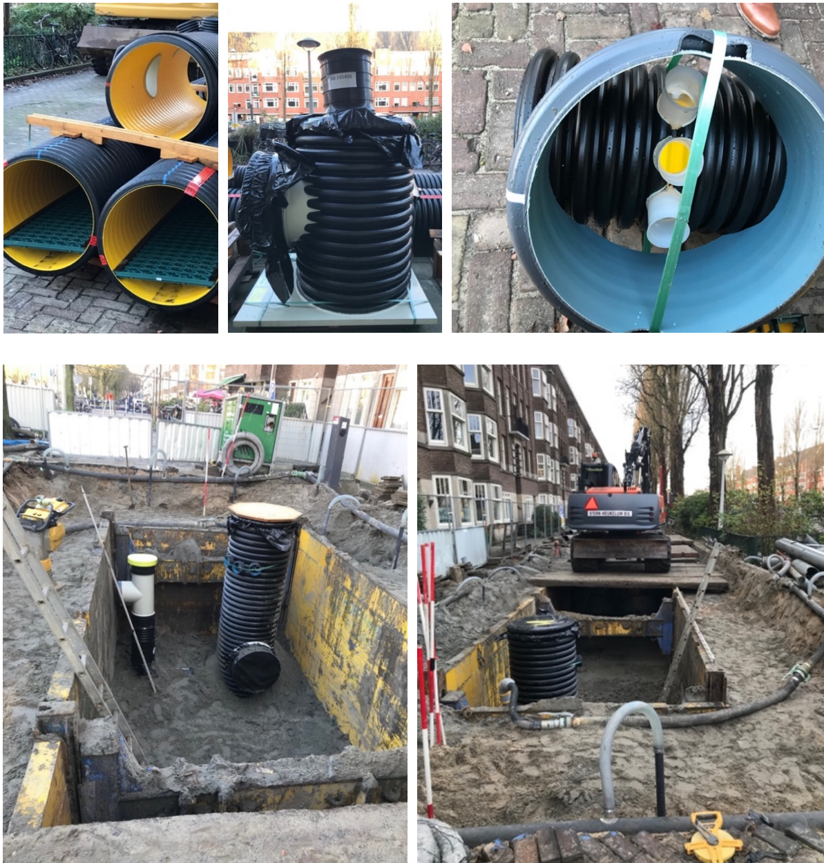
Figure C - 1: Installation of S4 on the Rooseveltlaan service road
