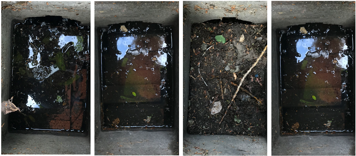
Figure C - 5: Gully pot check, with coarse sediments gathering
