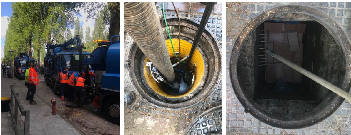
Figure C - 4: Cleaning S4 for the first time ( left, center ); filling manhole sinkers with bricks prior to start-up ( right )
