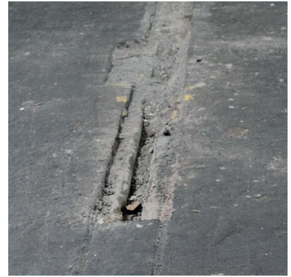
Expansion joint at the first floor where beams, columns and floors are separated. The space between the columns and floors is/is was covered.
