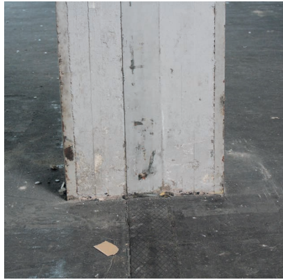
Expansion joint at the first floor where beams, columns and floors are separated. The space between the columns and floors is/is was covered.
