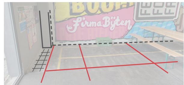
Stelcon plates (boundaries indicated with red), dimensions of 2x2m and 2x1.5m, placed between columns, space filled with pavers, walls built on top.
