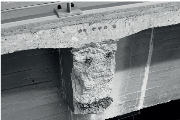
Cross section of a concrete beam and floor with reinforcement
