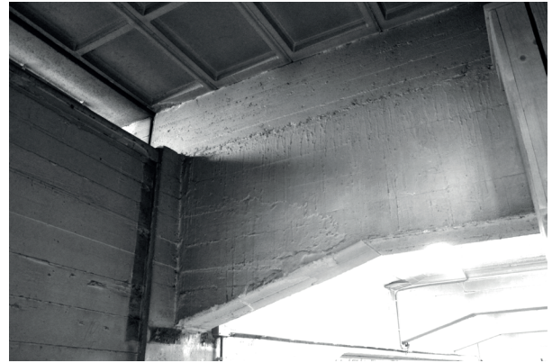
Junction where primary and secondary beam meet with the new roof element
