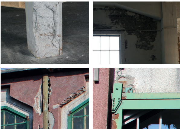
Spalling of columns, exfoliation of plaster and rust
