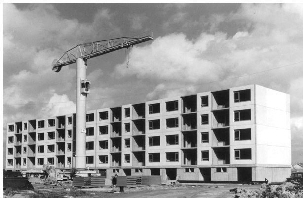
Fast assembly on site
