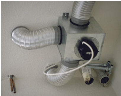
Figure 4. CMV unit for exhaust from kitchen, toilet and bathroom.
