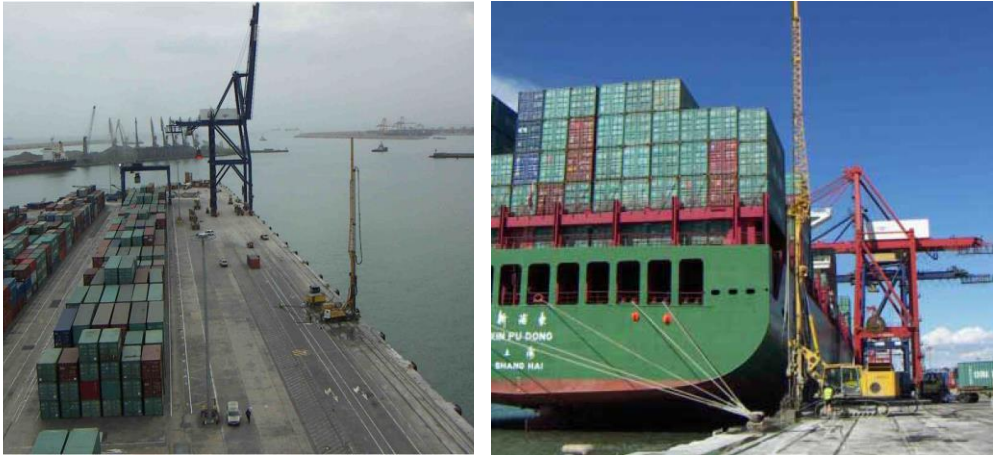
Figure 4-3 Super-jet grouting equipment operating at Port of Valencia (Fernández Vincent, 2008)
