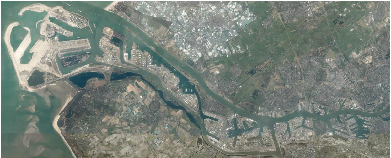
Figure 1-2 Satellite view of the Harbour Industrial Complex (Port of Rotterdam, 2014k)
