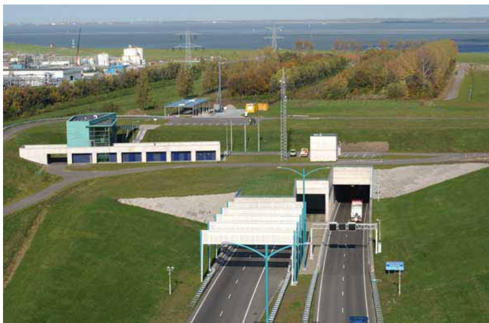
Figure 6.24 Entrance Westerschelde tunnel at Terneuzen
