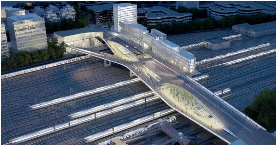
Figure 34 - Urban bridge that connects the two stations (Société du Grand Paris, 2024)
