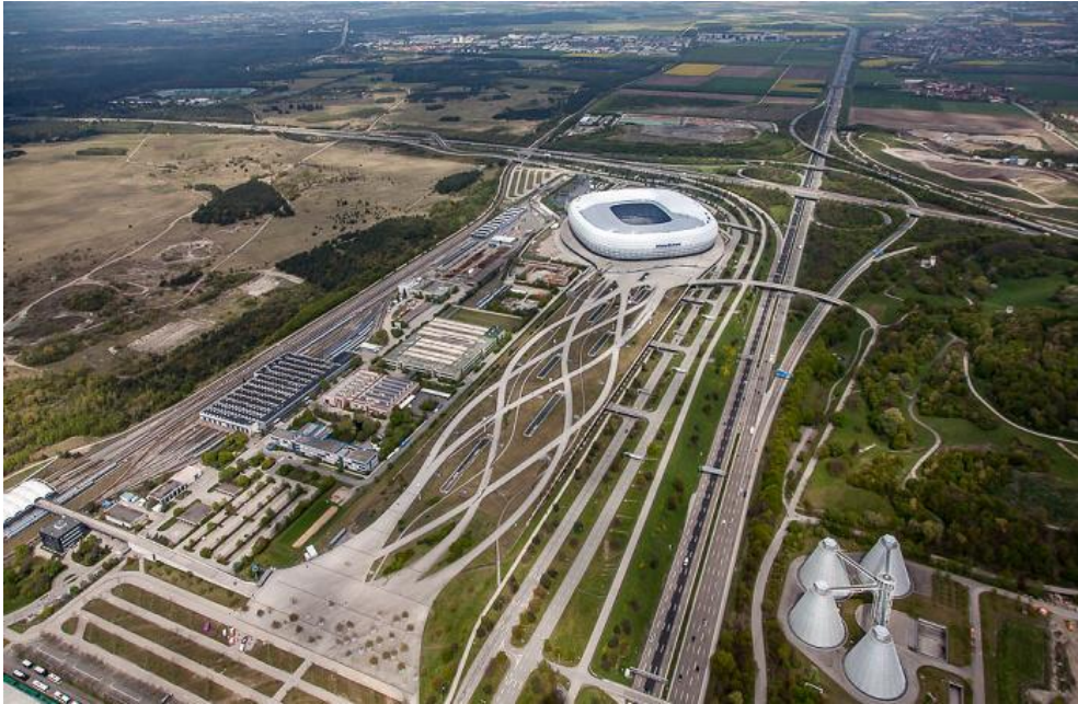
Figure 36 - Fröttmanning station (bottom-left) and the Esplanade towards the Allianz Arena
