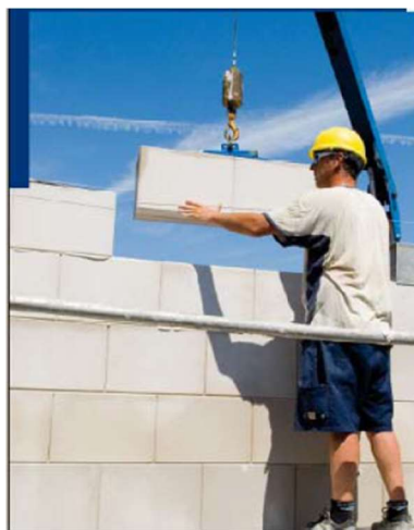
Figure 2.2 Building with CASIEL (Vermeltoort, 2008)
