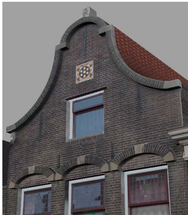
Figure 6.13 Special roof –and building design
