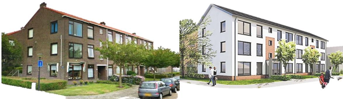
Figure 1. Before- and after depiction of the completed zero-energy pilot renovation of a block of 12 flats from 1951.
