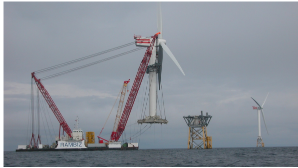
Figure B.6: Sheerleg crane Rambiz lifting a 5 MW turbine, from [134].
