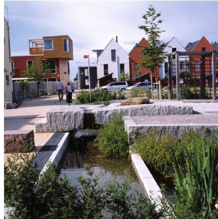
view inside the first block, looking south
