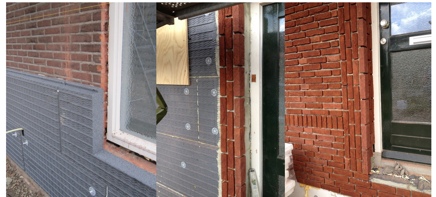
H 2 O renovation project with E-Board facade system by Vandersanden, Woningstichting Valburg (stedenbouwarchitectuur.nl, 2016)
