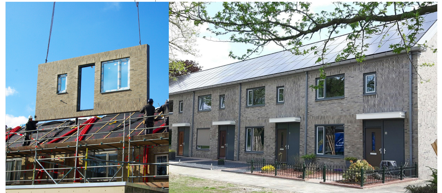
Placing prefab insulating elements (Knaapen, 2018)
