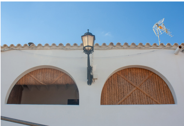
Figure 16: Manual blinds made from rush mats in El pozo de los Frailes (Almeria).
