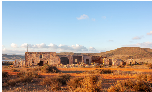
Figure 9: South facade of an old farmhouse in Nijar (Almeria).
