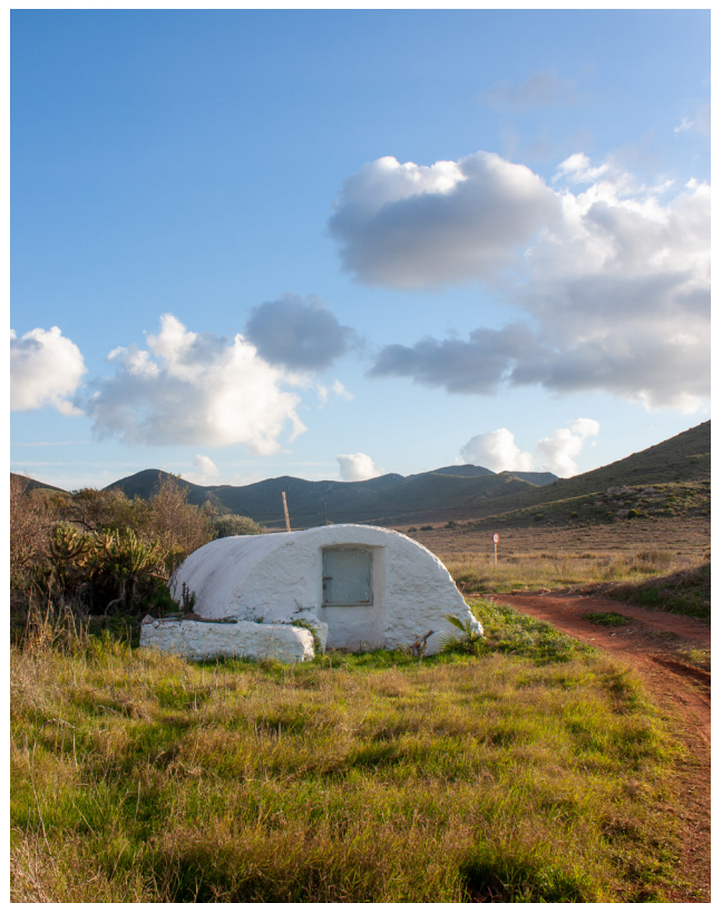
Figure 2: Water cister "Aljibe" in Cabo de Gata (Almeria).
