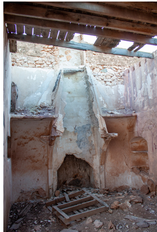
Figure 21: Chimney in an old Cortijo in Nijar (Almeria).
