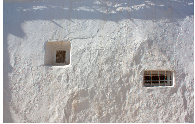
Figure 12: Facade in Nijar (Almeria).
