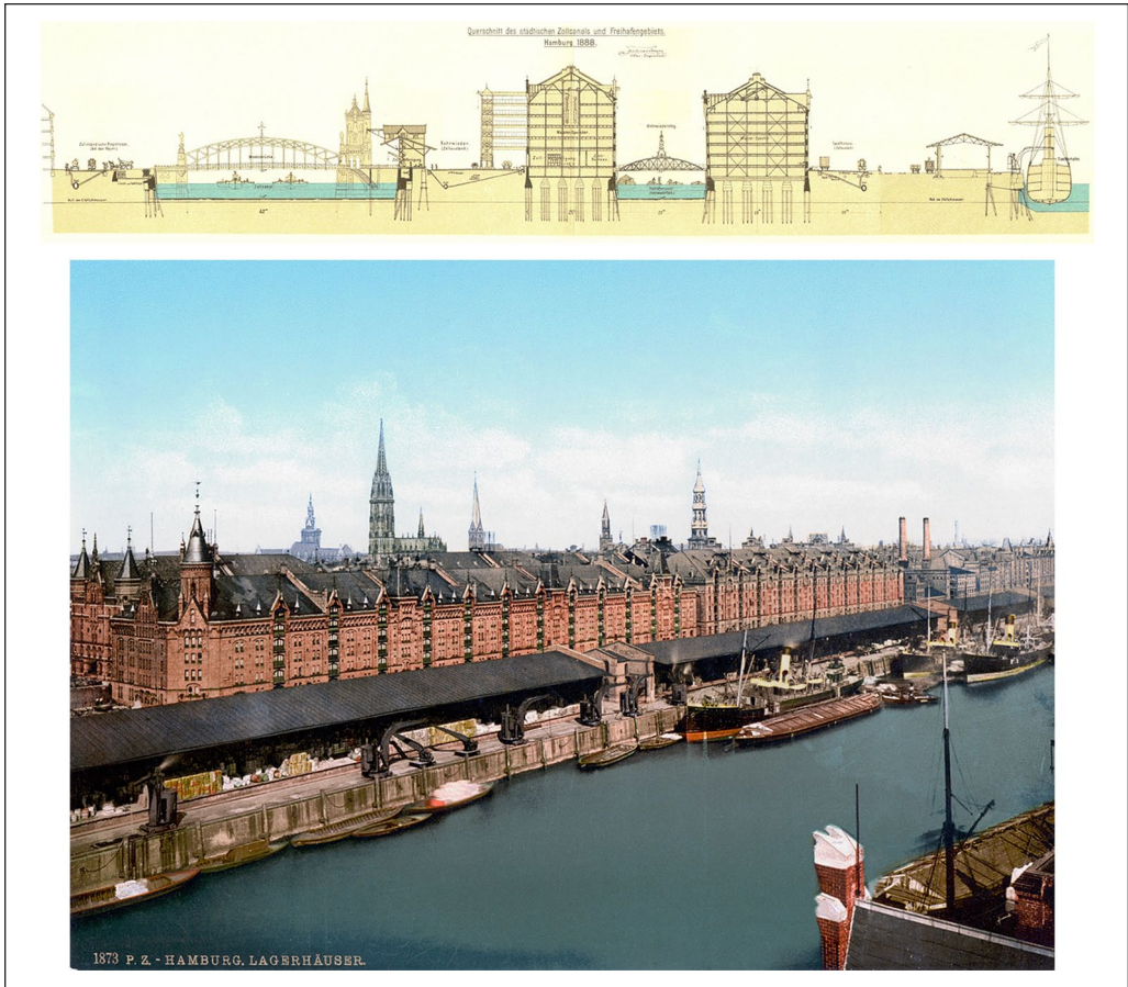
Figure 8. Section of the Speicherstadt in Hamburg in 1888 and photo of 1890 with the Sandtorhafen from 1873, Planned by Oberingenieur Franz Andreas Meyer (1837-1901) —Aus dem Hamburger Freihafengebiet, Hamburg 1888, Strumper & Co.
