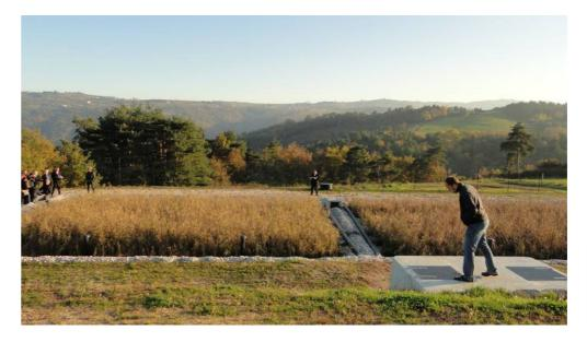
Fist stage of the French System for wastewater treatment.
