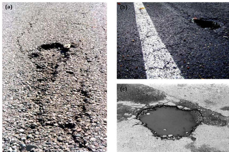
Figure 1.2. Deteriorated pavements due to water induced damage: (a) ravelling caused by segregation; (b) and (c) pothole formation (reprinted from Pavement Interactive http://www.pavementinteractive.org/ ).
