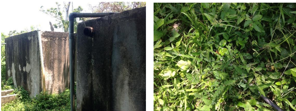
Figure 25: Storage tanks (right) and unauthorized connections (left).
