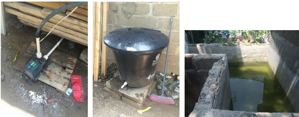
Figure 34: 1/2" water pump (left), 250L plastic water storage tank (middle) and constructed water storage (commonly known as 'alberca') (left).
