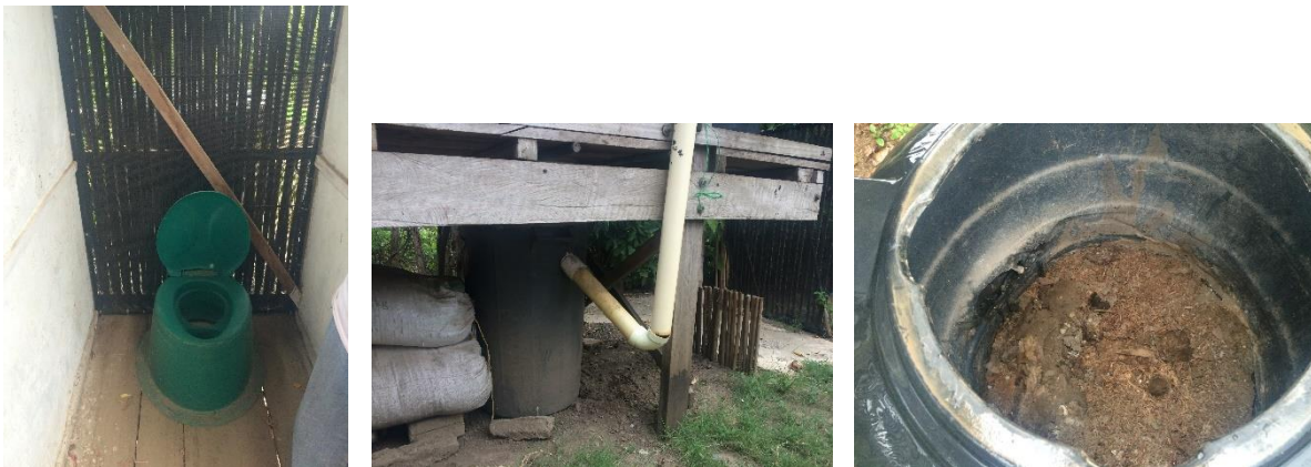
Figure 33: Juan's dry toilet. Toilet base (right), aeration tube and storage tank (middle), compost base (left).
