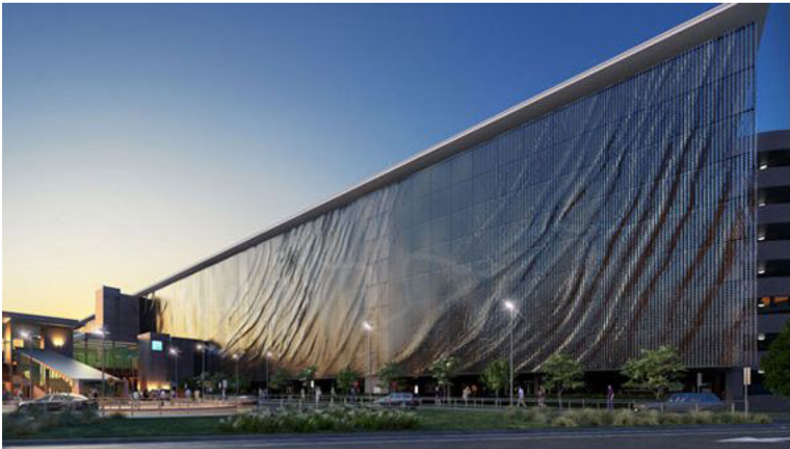
Reference Ned Kahn facade https://nedkahn.com/portfolio-category/wind
