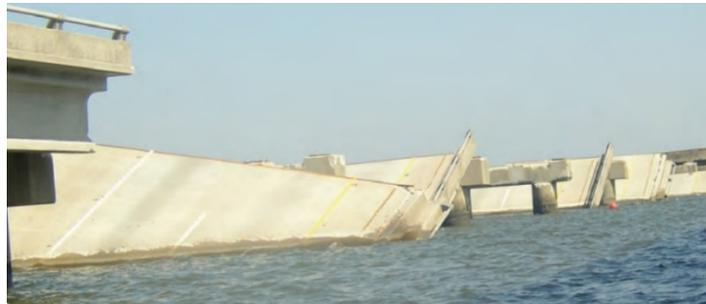
Figure 2- 17 Total displacement of spans. One end of span in the water, another side on the bent cap beam [26].
