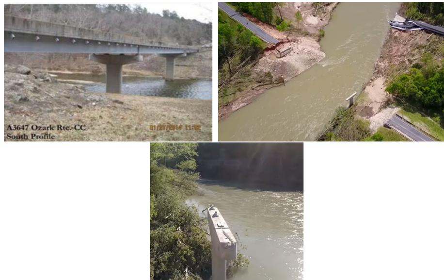
Figure 2- 16 Hammond Bridge before 2017 flood (left) [22], Hammond Bridge after the flood(middle), Lack of damage to the leading side of the pier cap and presence of damage and scratch on the trailing side(right) [23].
