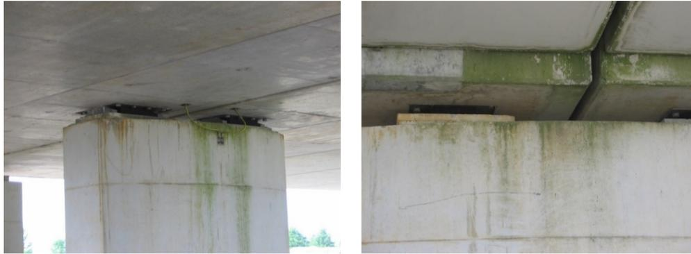
Figure 4- 35 Example of elastomeric bearing between bridge pier and deck [38].
