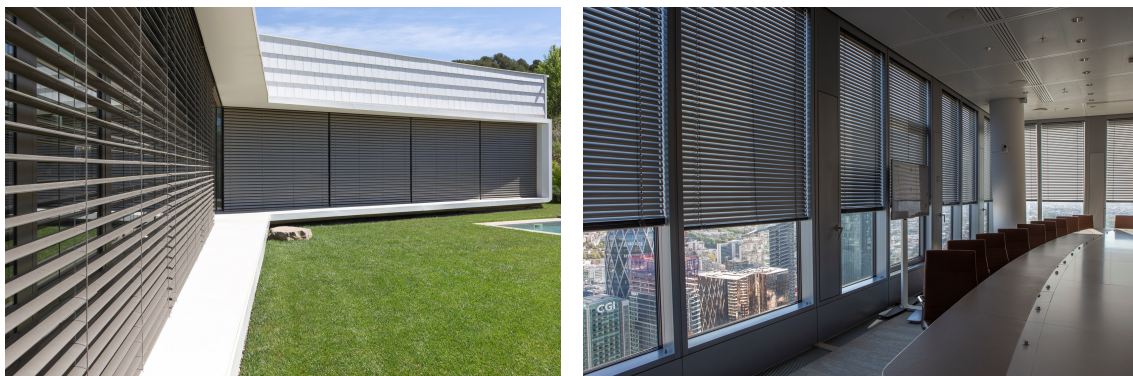
(a) External Venetian blinds.
