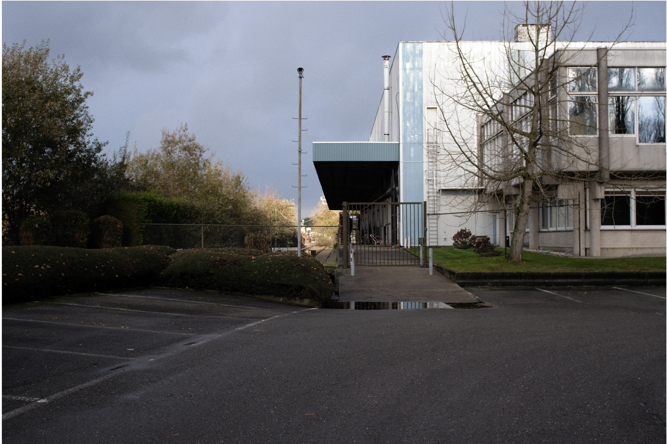
backside railway tracks
