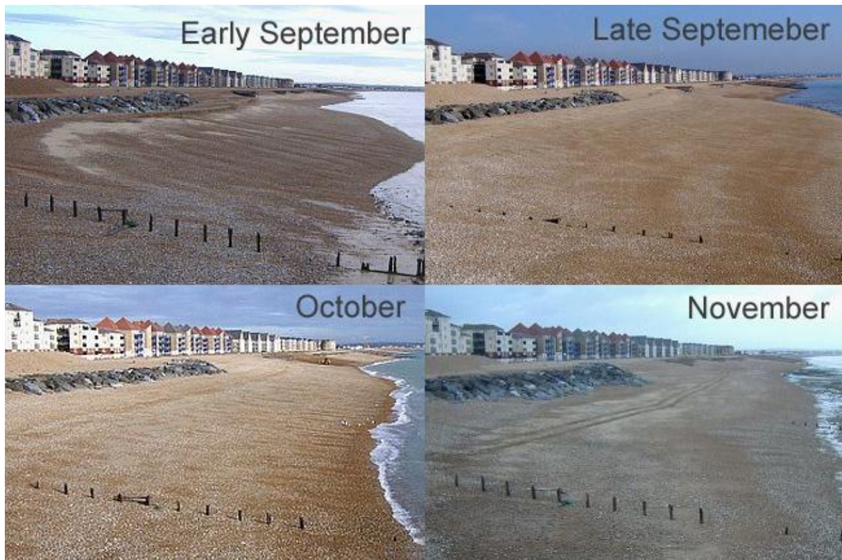
Figure 13: Shingle replacement in Pevensey Bay. Source: http://www.pevensey-bay.co.uk/recharge.html 2
