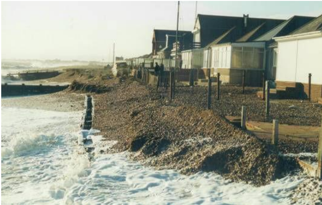
Figure 12:Typical erosion prior to improvement works; source: Thomas and Amies (2009)
