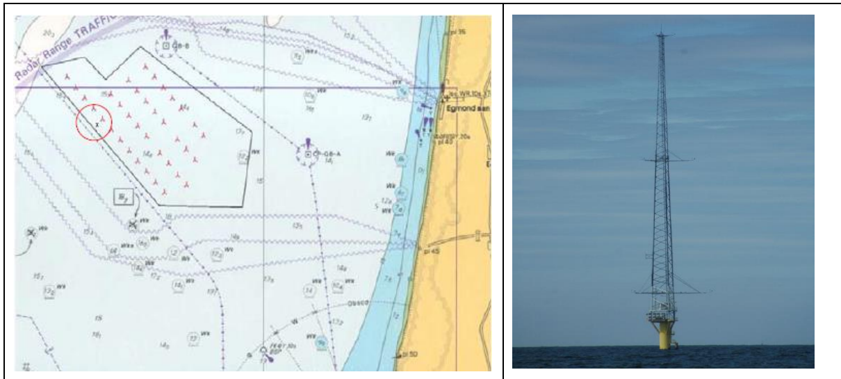
Figure 2: The OWEZ site location and the meteorological mast shown with a red circle on the map. Ref. [5]
