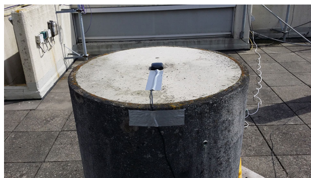
Fig. 2 u-blox M8T patch antenna placed on concrete pillar at the TU Delft GNSS observatory on top of the NMI building in Delft
