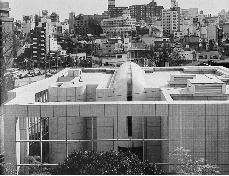
Figure 20. Exterior Shoto Club (Ohashi, 1988, p. 29)
