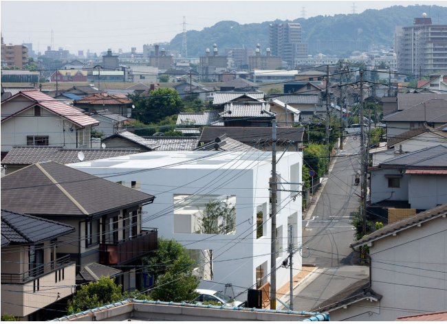
Figure 30. Exterior House N (Baan, 2008b)
