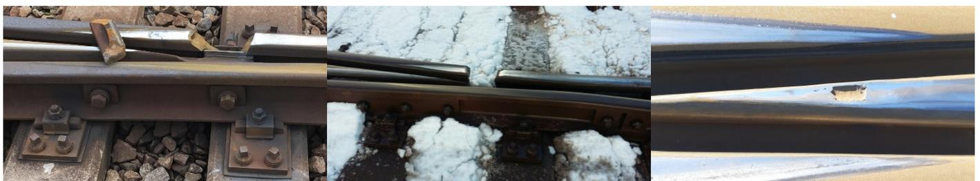
Figure 4 - Examples of damaged crossings [1]
