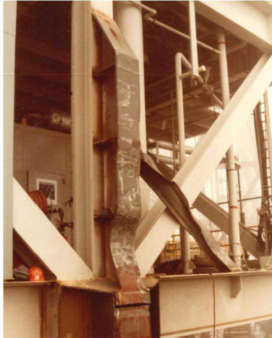
Figure 1.2: Example of damaged bumper
