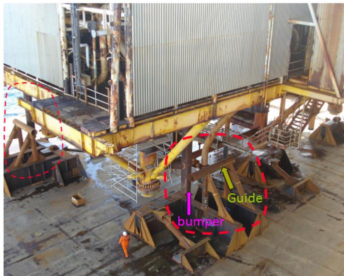
Figure 1.1: Example of reverse installation module on barge with guides
