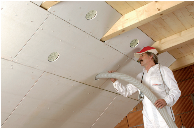
Image 6.21: Filling cavities with cellulose insulation
