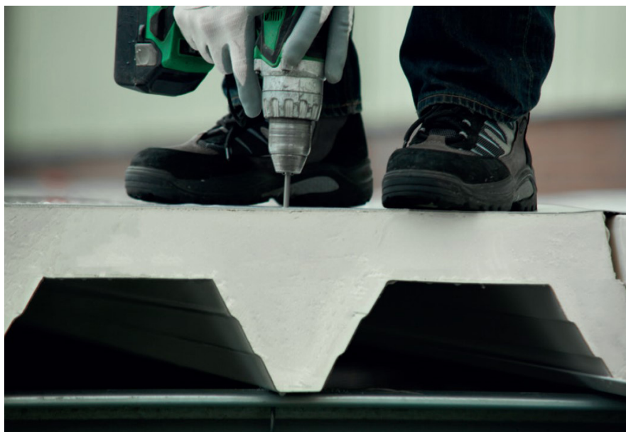
Image 4.12: Kingspan X-dek 106 sandwich panel being installed
