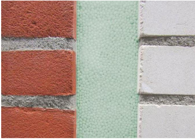
Image 3.03 & 3.04 : Biofoam: PLA based rigid insulation foam
