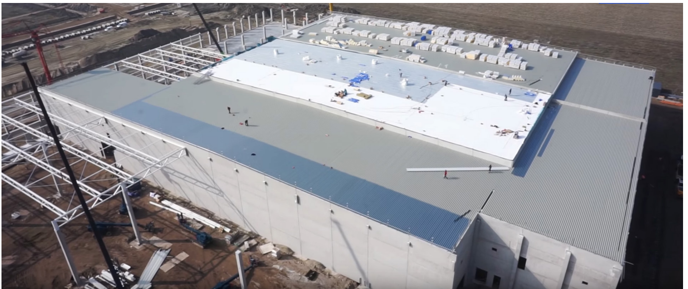
Image 3.12: Men on top of DC during construction, applying insulation manually
