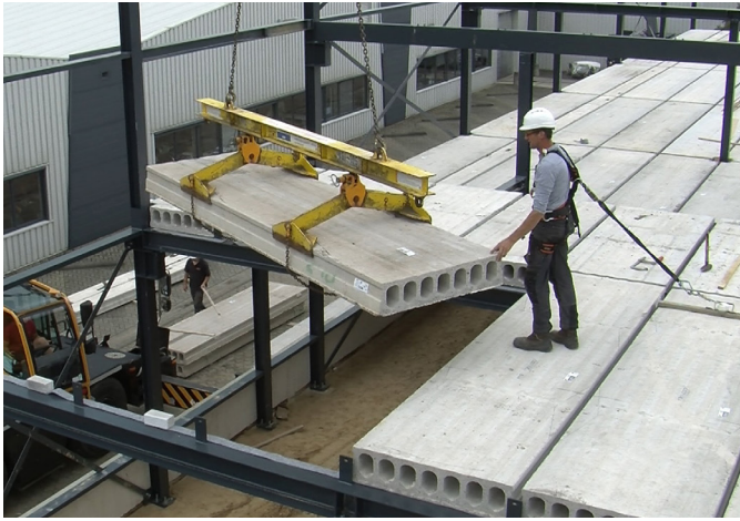
Image 5.71: Hollow core slabs floors being installed
