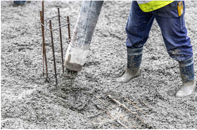
Image 6.20: Pouring concrete
