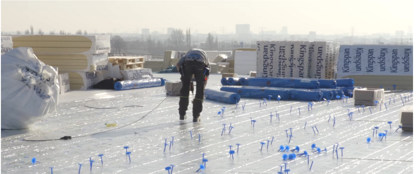
Image 3.11: Foam isolation being applied on DC, manually in blocks
