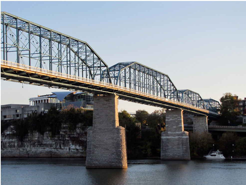
Figure 5.7: The Walnut Street Bridge uses a steel truss to connect the center of Chattanooga, TN with the North Shore
