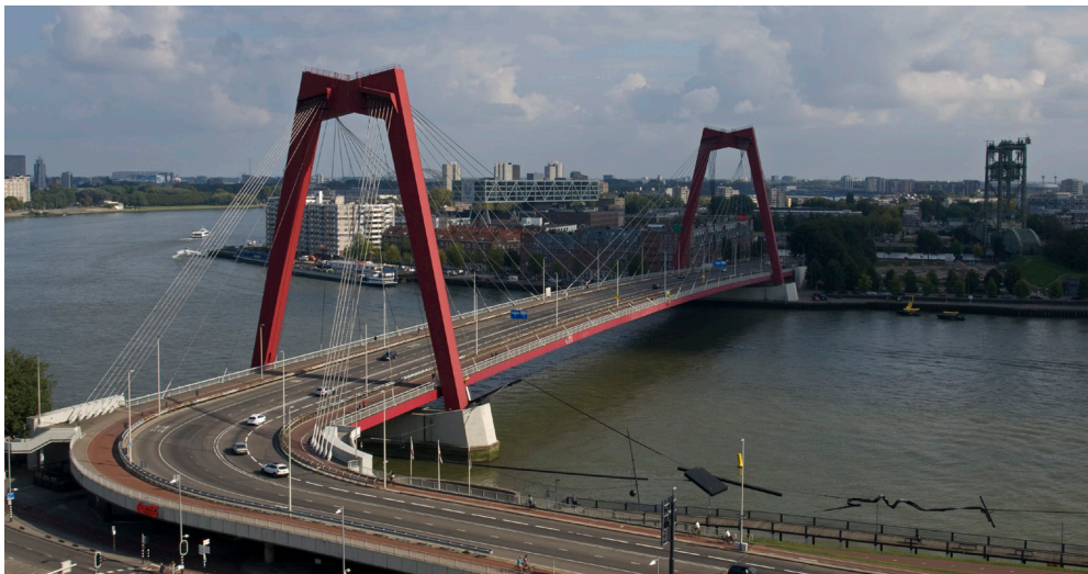
Figure 3.9: A view of the Willemsbrug crossing the Nieuwe Maas river in the city of Rotterdam as seen from the North (photo: Flickr)
