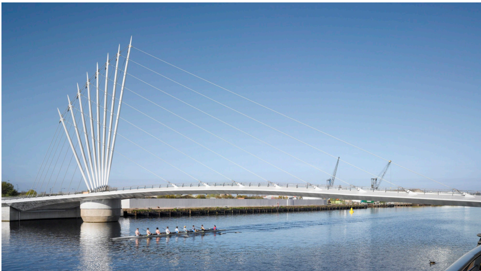
Figure 5.28: The Media City Footbridge is an asymmetrical swing bridge across the Manchester Ship Canal in Manchester (Wikimedia Commons, 2014)
