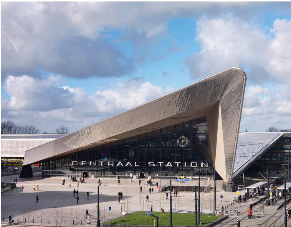
Figure 3.2: The newly developed area in front of the Central Station in Rotterdam (Nationale Staalprijs, 2014)
