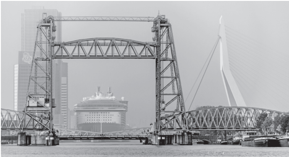
Figure 4.5: An aerial view of the Lloyd pier in the north of the location (Google Maps, 2017)
