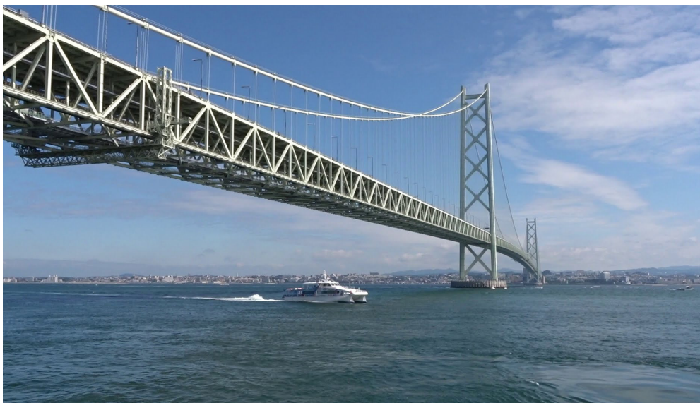
Figure 5.18: The Akashi-Kaikyo Bridge is a suspension bridge with the largest main span in the world and crosses the Akashi strait near Kobe, Japan (Wikimedia Commons, 2015)
