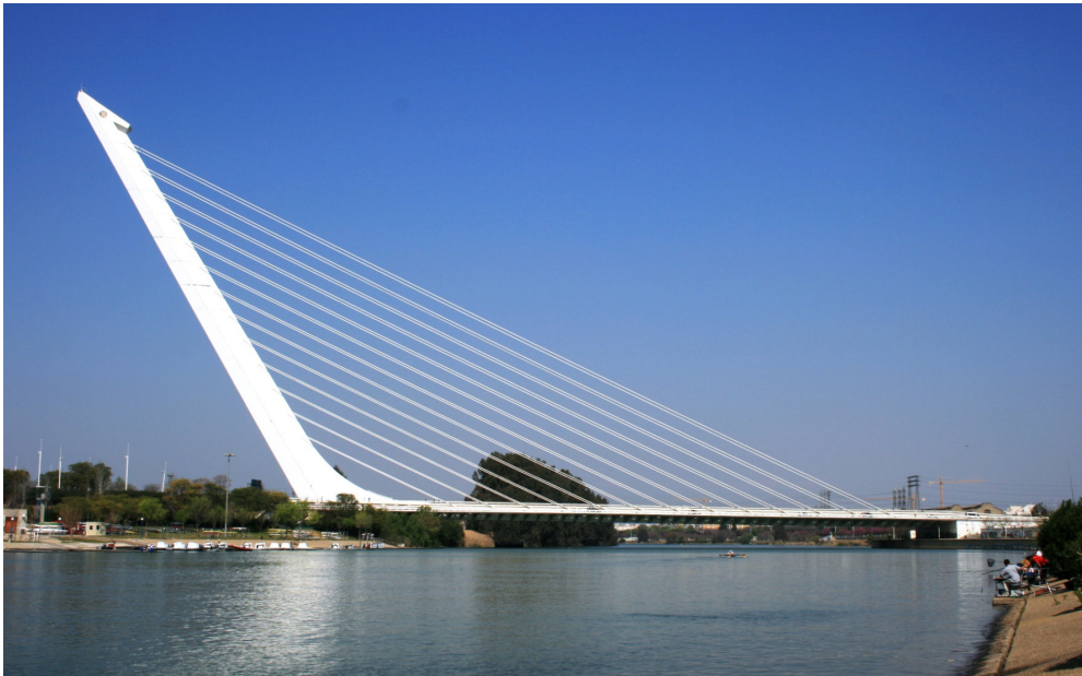
Figure 5.21: The Alamillo Bridge in Seville crosses the Guadalquivir river in Seville, Spain (Wikimedia Commons, 2015)
