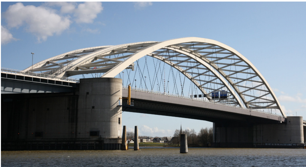
Figure 3.12: A view of the van Brienoordbrug crossing the Nieuwe Maas river east of the city of Rotterdam as seen from the North (photo: Flickr)
