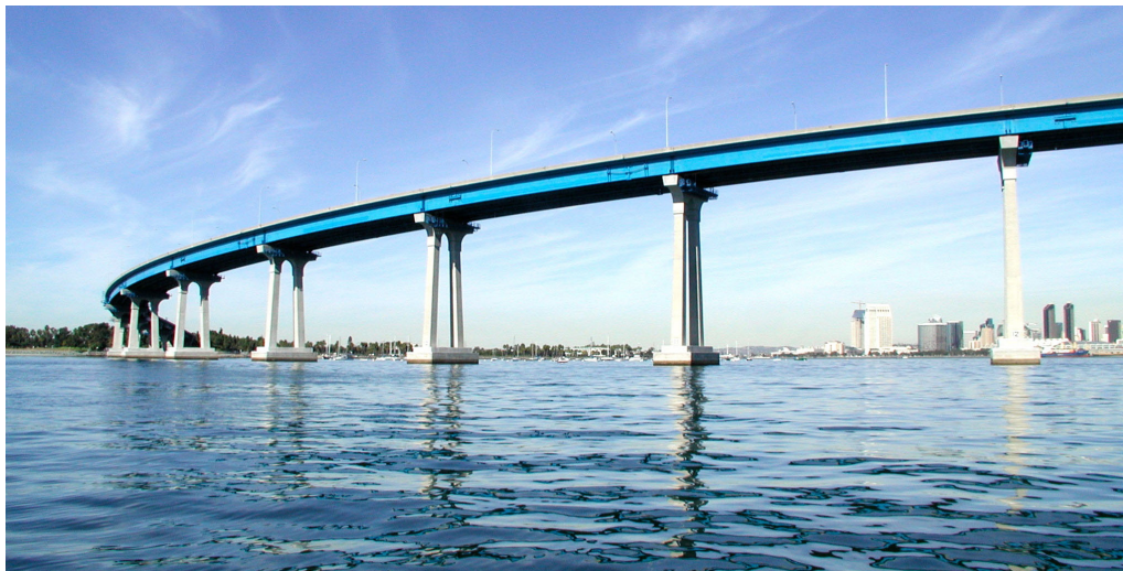
Figure 5.3: The Coronado Bridge in San Diego, CA is a beam bridge which uses concrete and steel girders to cross the San Diego Bay.
