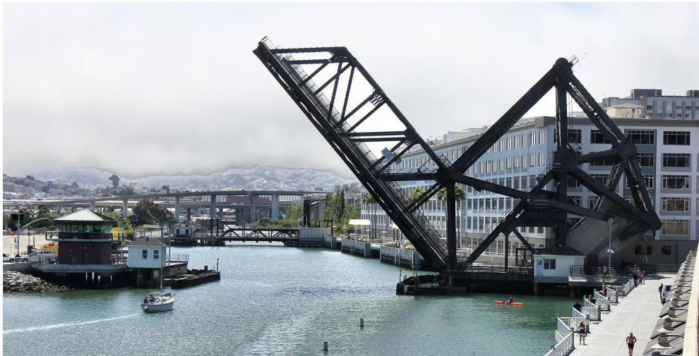
Figure 5.24: The Lefty O'Doul Bridge is a drawbridge connecting China Basin and Mission Bay in San Francisco, CA (Wikimedia Commons, 2015)
