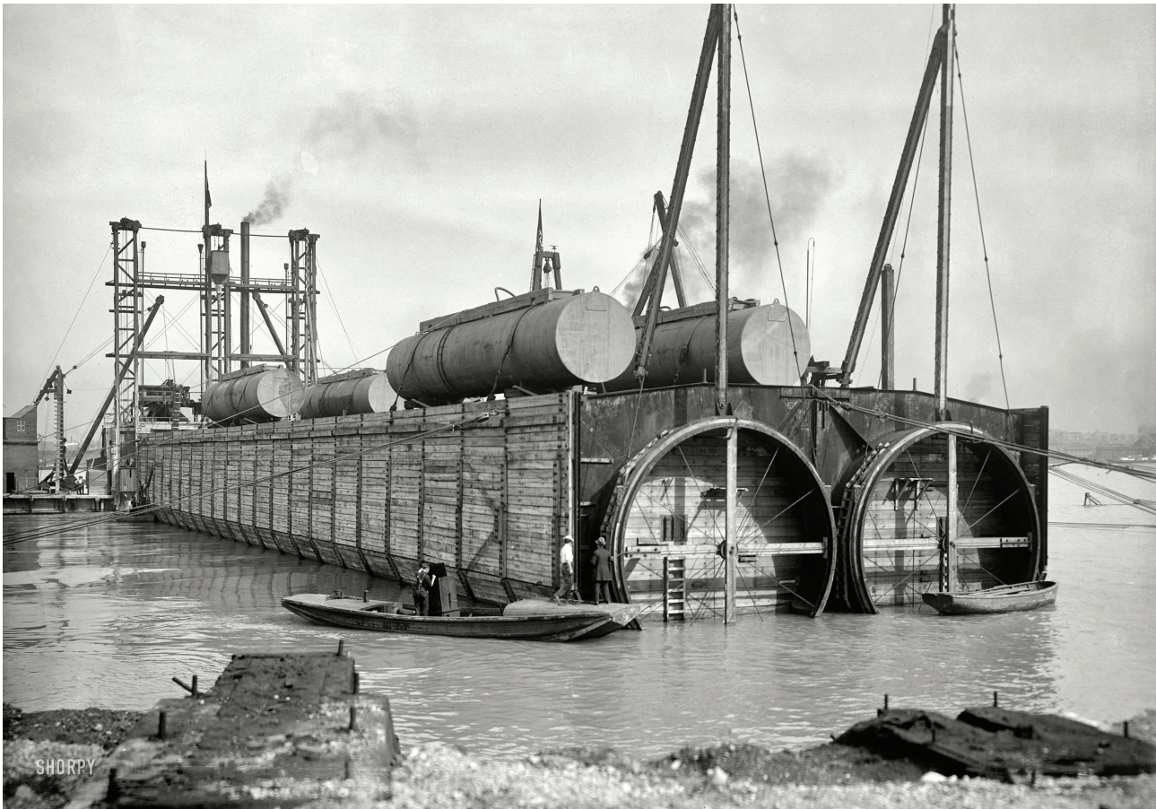
Fig. 13: Section of the Detroit River tunnel in 1910
