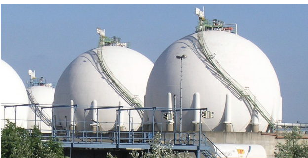
Fig. 05: Petroleum refinery, Karlsruhe
