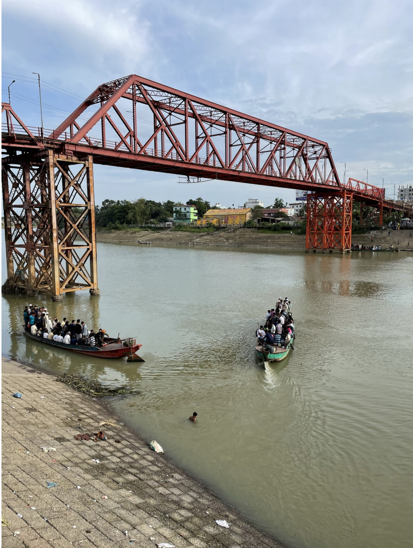
Kean bridge, Sylhet Source: Own photograph
