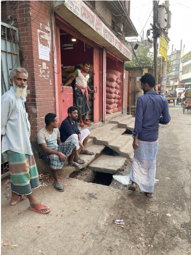
Open sewage in Old Dhaka Source: Own photograph
