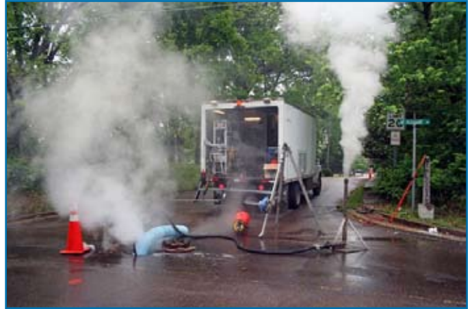
Figure 31: A CIPP liner has been inserted from a manhole and is now being cured (AOC Resins)
