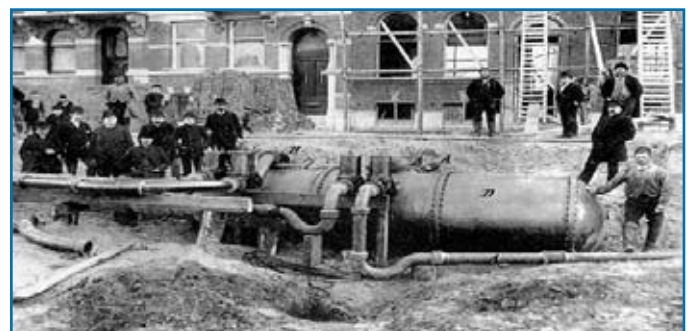
Figure 7: Construction of a Liernur system
