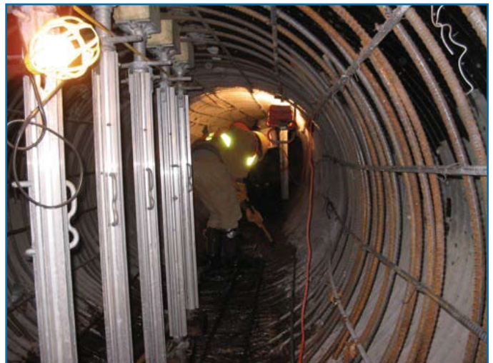
Figure 32: Shotcrete (sprayed concrete) lining applied to a corrugated steel sewer pipe in Ottawa, Canada (Environmental Science & Engineering Magazine)
