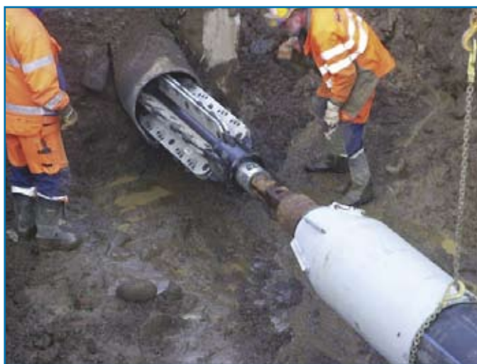
Figure 25: Pipe-cracking, clearly showing the new pipe section attached to the rear of the crack-head (Trenchless Australasia)
