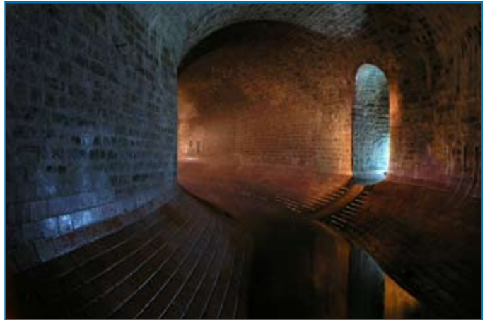
Figure 1: Victorian sewer underneath London ( http://www.flickr.com/photos/jondoe_264 )
