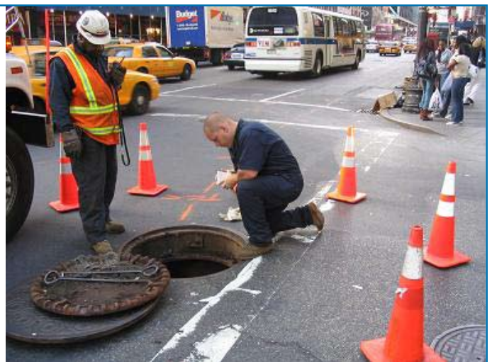
Figure 37: Sewer works in dense urban environments can result in heavy traffic disruption
