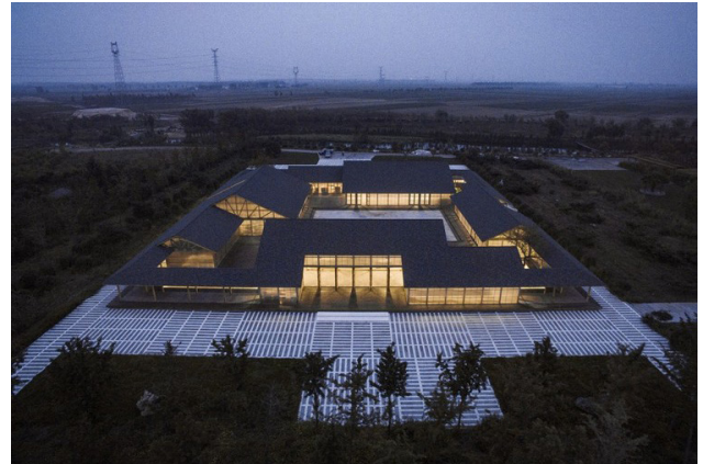
Figure 08 | An organic food factory in Tangshan, China. It is in a traditional Chinese architectural style, owning a corridor and a courtyard as the hub for production. The application of modern material, creating a cozy working atmosphere increase the spatial quality of usual productive architecture.
