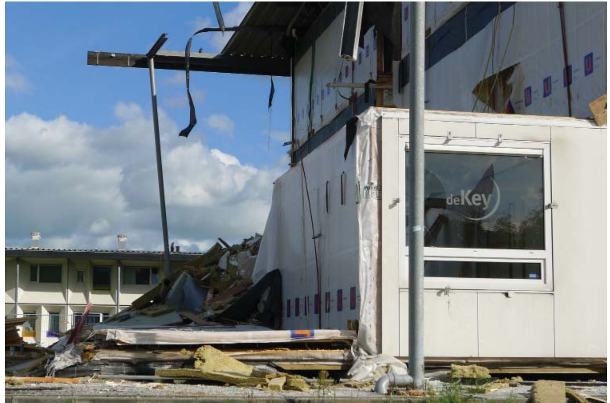
Demolition of temporary student housing in Houthaven. (own picture)
