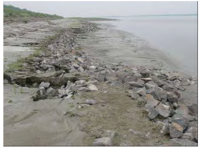
(b) Damaged section with shifted rock with exposed geotextile and some sand deposits
