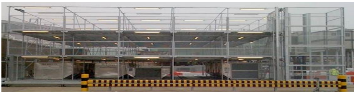
Figure 23 Triple deck empty container storage (Laxmi Engineering, n.d.)
