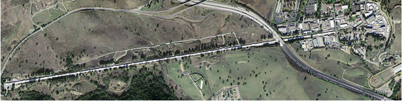
Figure 2.5: Aerial photo of the SLAC National Accelerator Laboratory, with detector complex at the right (East) side
