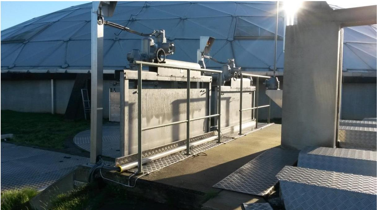
**Fig B.2.** Picture of the controllable valves to dynamically operate the PCs in the Primary Clarifier Control
