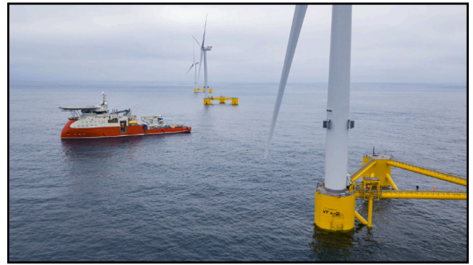
Fig. 1. Support vessel and wind turbine, respectively a planar and tubular maritime structure.
