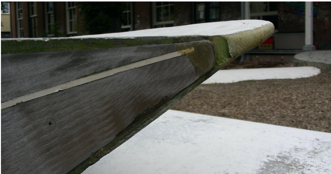
Figure 12. Brittle edge of a blade, sharp on the top-right part of the picture, where the epoxy resin and the glass fibres are damaged (Photo by Piero Medici, 2011).
